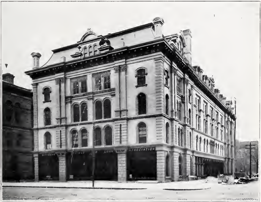
Case hall, corner Superior street and Wood (East 3rd) street. Built, 1866-7. As it looked just before it was torn down, 1901-2, to make room for new postoffice.
